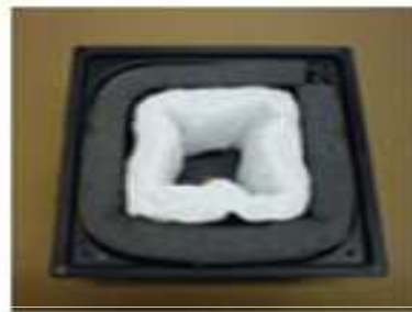
Fig.2 Install 3M foam and a coustic insulation.
