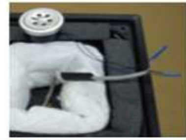
Fig.4 Secure connections with connectors.
